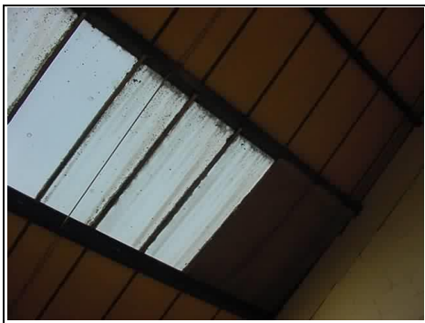
Close up of the GWPP (Georgian Wire Polished Plate)
