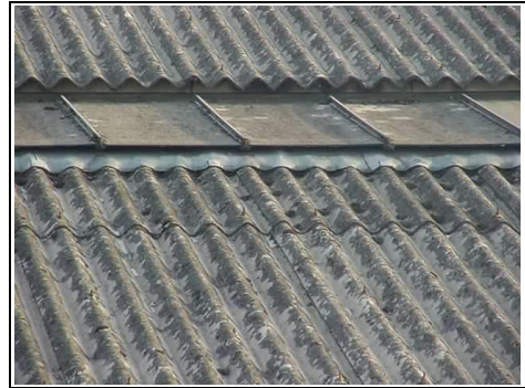
External view of roof lights
