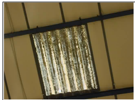
GRP (glass reinforced plastic) window, they are not always metal and they are not always glass!
