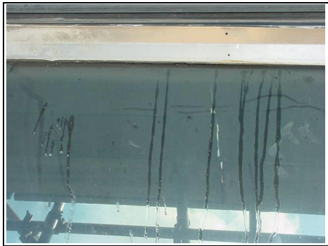
Leaking window
