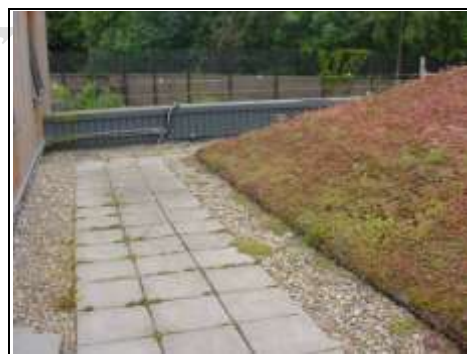
Example of pavia slab on flat area next to a living roof
