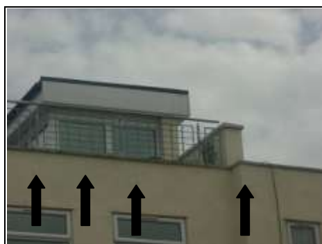
Weep holes in parapet wall
