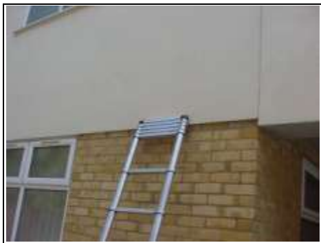
Drip detail to base of render
