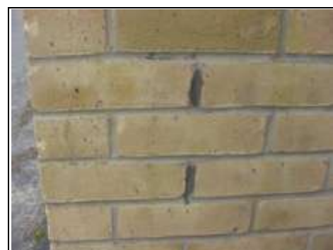
Two repointed perpendicular ends to the brickwork (perp ends)
