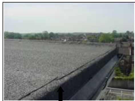
Looking at the felt roof itself, showing uneven cuts and rucking to upstand
