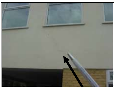
Vertical cracking to front
