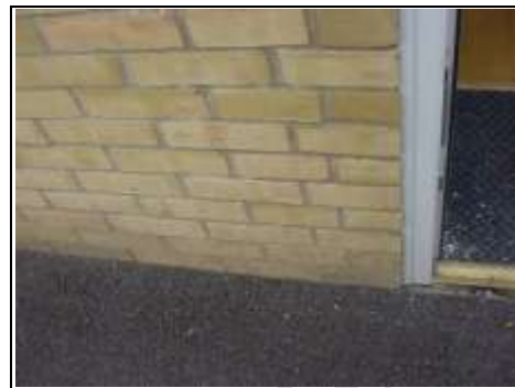
Stretcher bond brickwork
