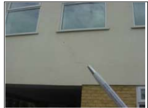
Cracking to the front of the property
