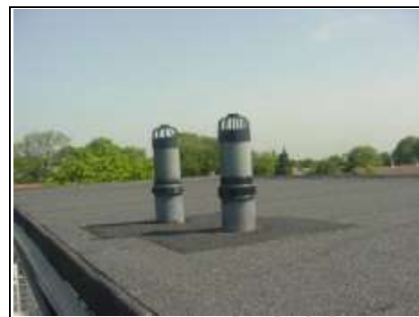
Soil and vent pipes
