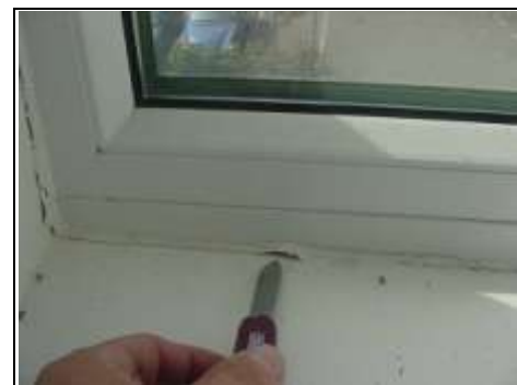
Dampness meaning that the mastic around the windows is coming out
