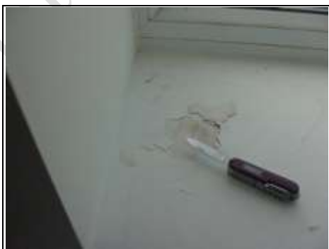
Flaking paint on window sills – we saw condensation
