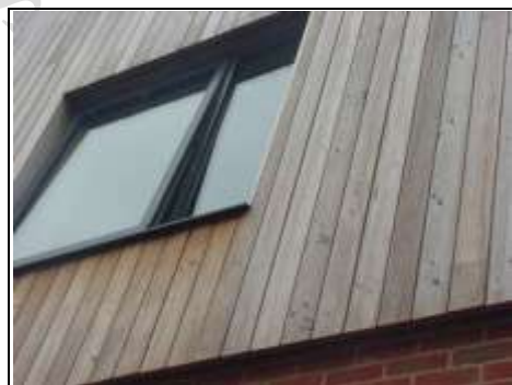
Example of timber rain cladding on another building giving protective layer to blockwork beneath
