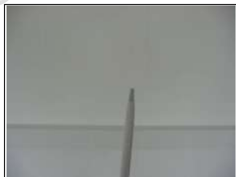
Further hairline cracks
