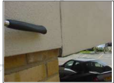
Testing the condition of the render
