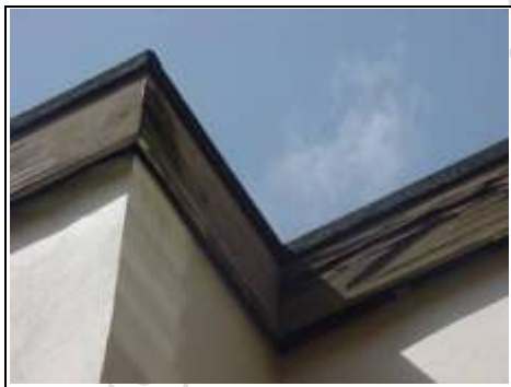
Deteriorating fascia board
