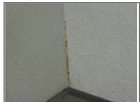
Wrong angle beads have been used in some areas
