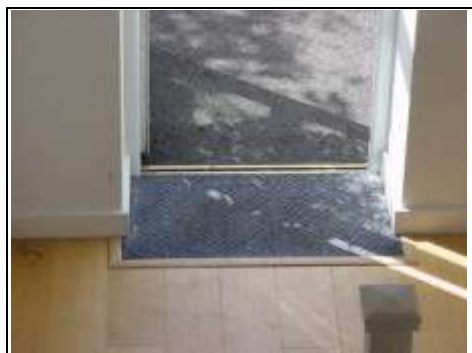
Threshold to front of property is— nearly same height as the outside floor
