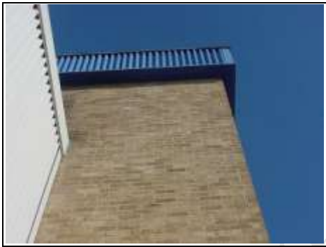
Fascia and soffit cladding
