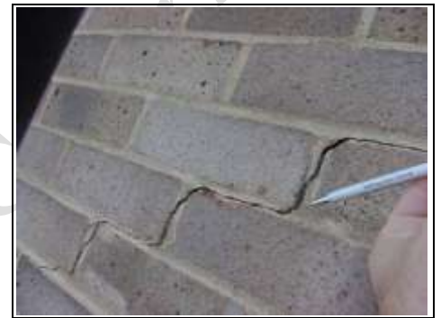
Cracking to left hand side
