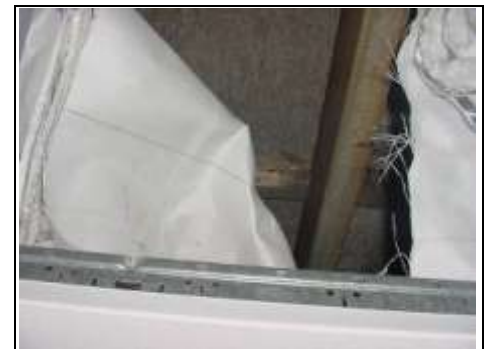
Firefly Plus paper that isn't fitted properly
