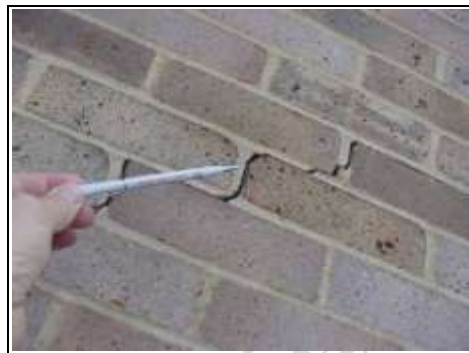
Cracking to brickwork
