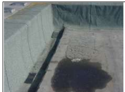
Ponding to the roof indicating low areas. Also crocodiling/crazing visible to the surface of the bitumen repair
