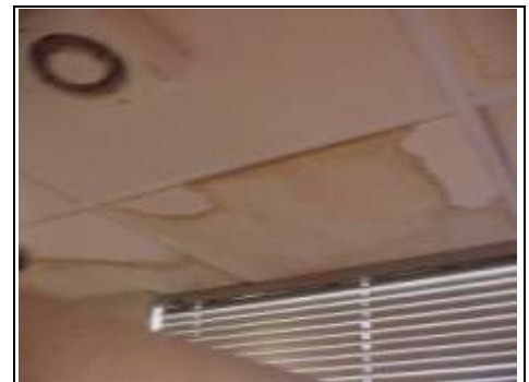
Water staining in gents toilets
