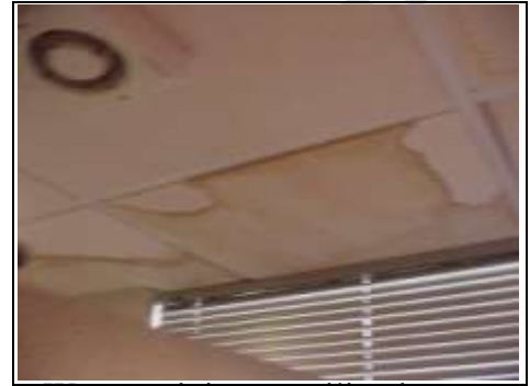
Water staining to ceiling in gents toilets
