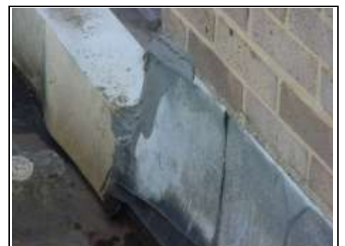
Old repairs to guttering
