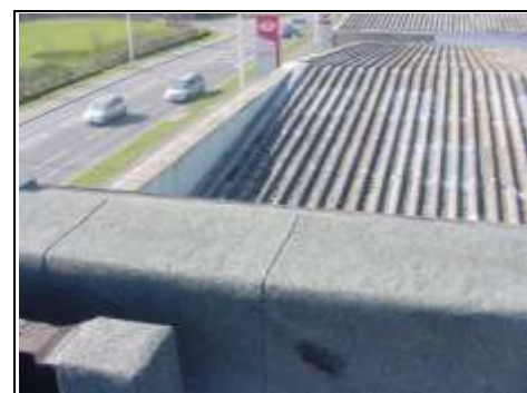
Asbestos Roof
