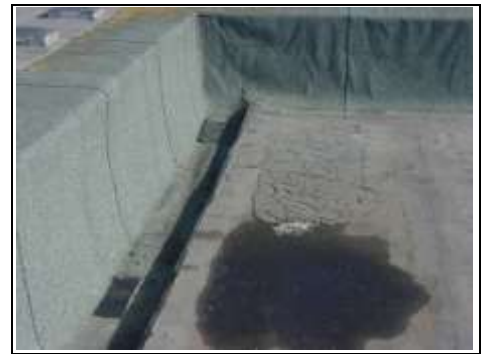
Ponding to roof
