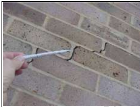
Cracking to left hand side
