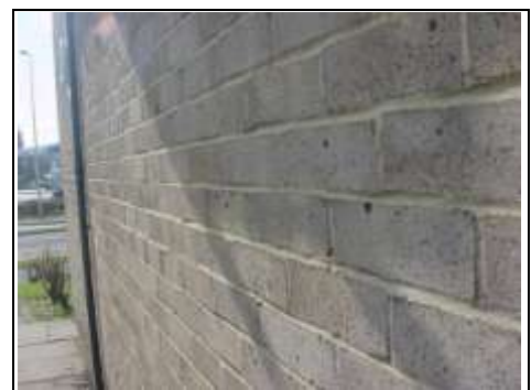
Stretcher bond brickwork
