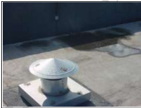
Ponding to roof
