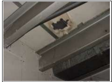
Water leak in store cupboard
