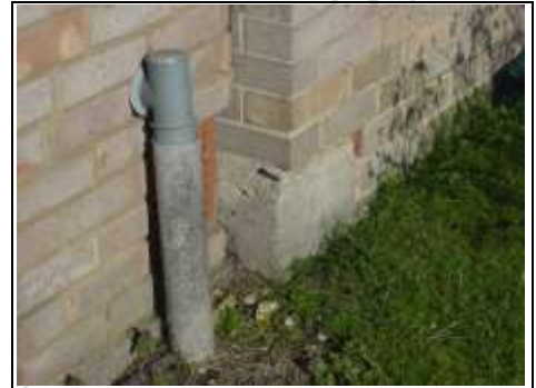
Foundation visible at bottom of brickwork
