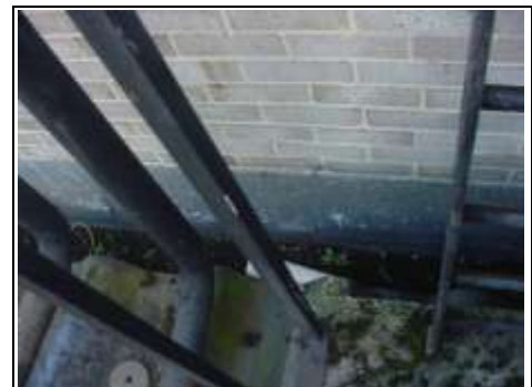
Blocked box gutter
